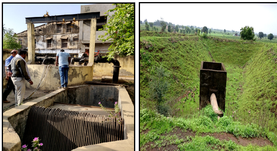
Fig.15 & 16: Nalla interception & Pumping Station
